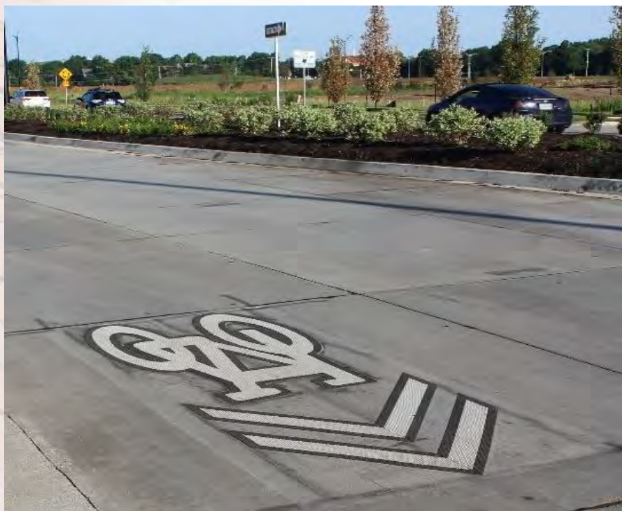
Shared-Use Pavement Markings
