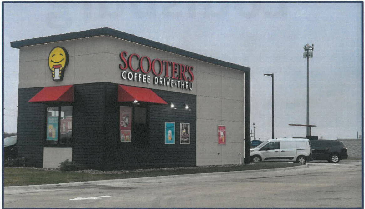
Scooter's Coffee, 1502 West Amity St. – Construction Completed 2025
