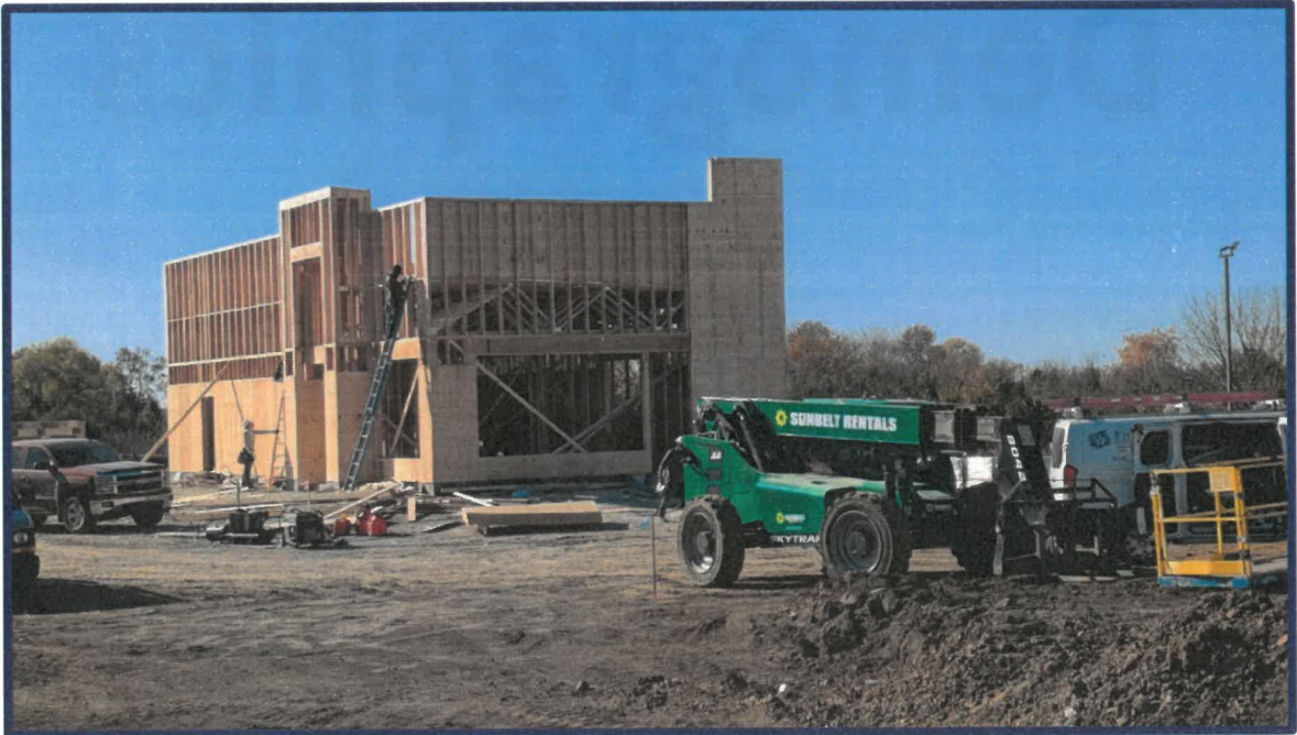
Taco Bell, 1401 West Amity St. – Under Construction 2025
