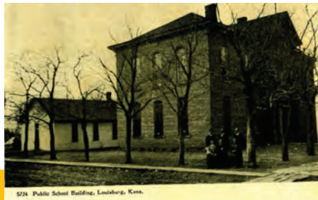
574 Public School Building, Louisburg, Kans.
