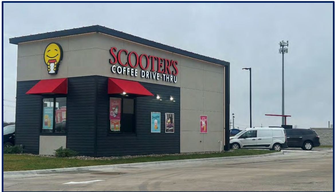
Scooter's Coffee, 1502 West Amity St. – Construction Completed 2025
