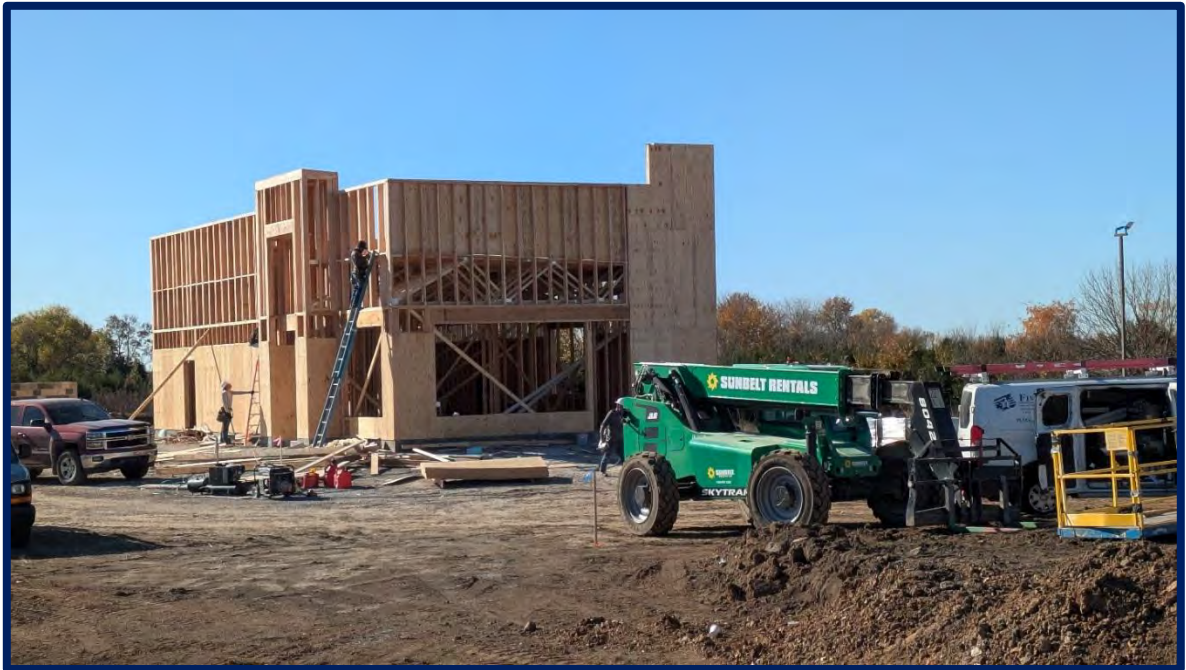
Taco Bell, 1401 West Amity St. – Under Construction 2025
