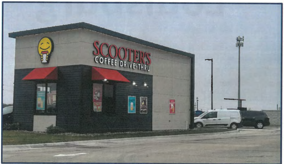
Scooter's Coffee, 1502 West Amity St. – Construction Completed 2025
