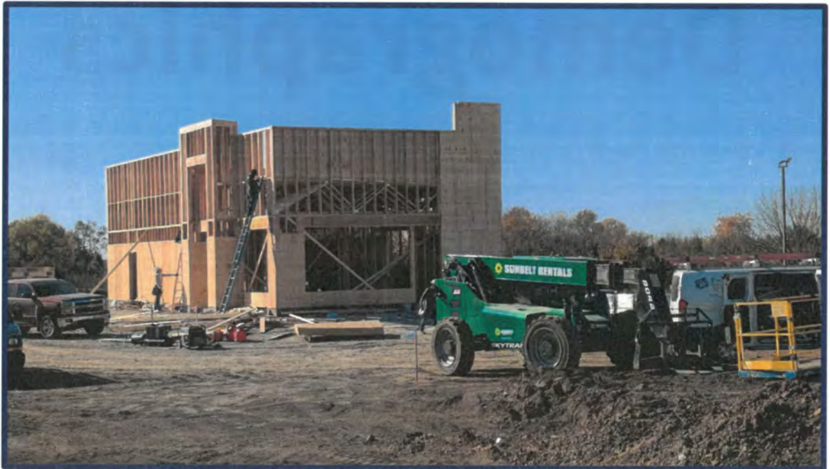
Taco Bell, 1401 West Amity St. – Under Construction 2025
